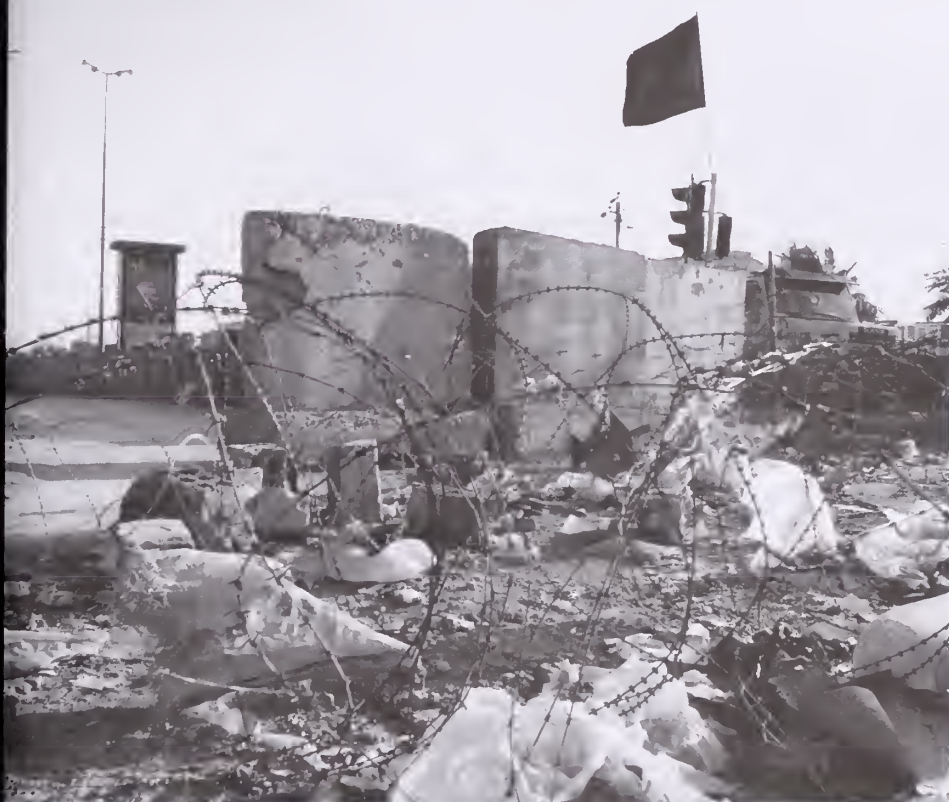
Blast walls are everywhere in Baghdad, and provide protection against explosions. They are usually found surrounding military installations, hotels and NGO offices. Baghdad, Iraq. March 21, 2004. ©Andrew Stern / AndrewStern.net
