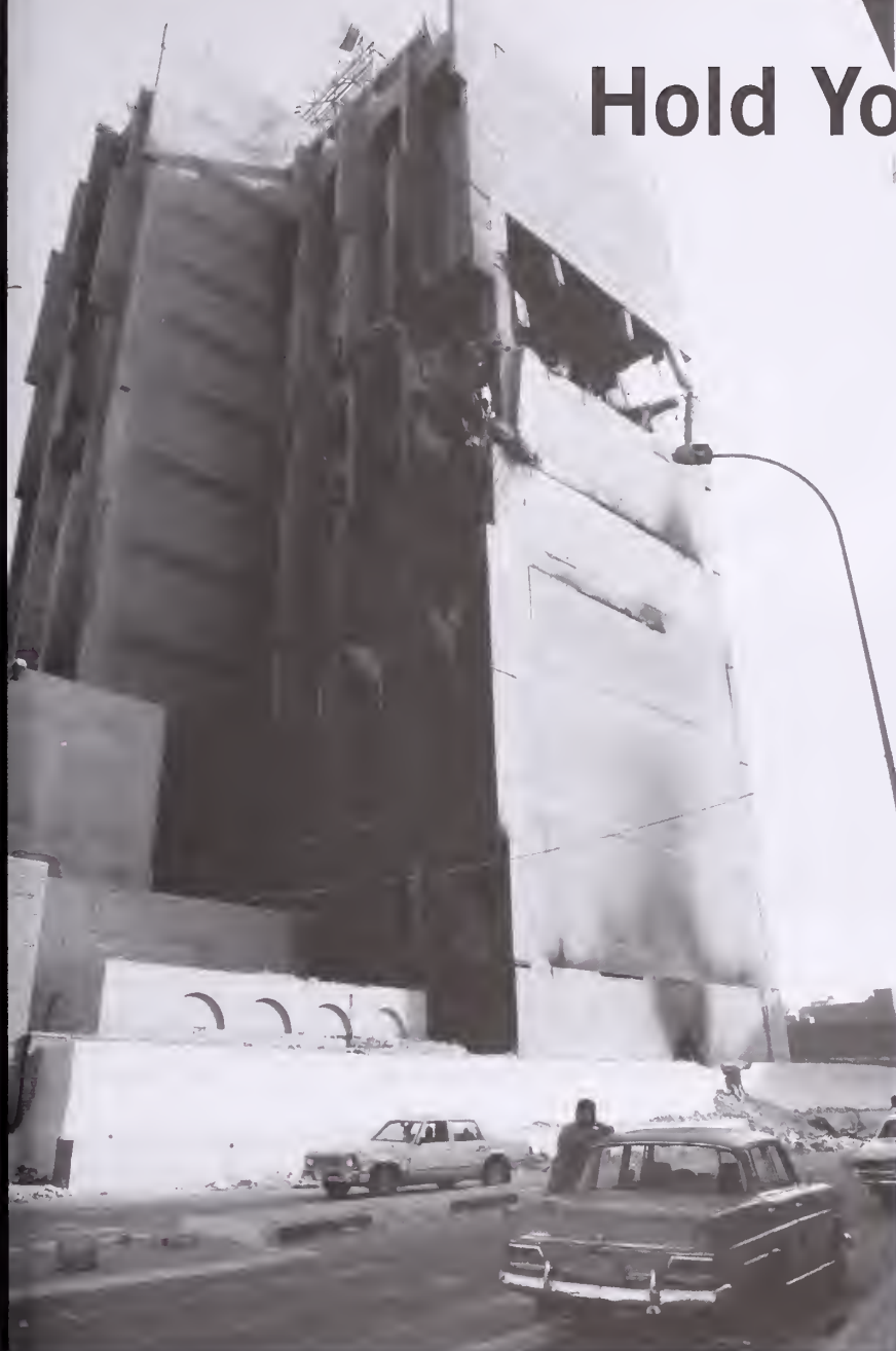
A telecommunications center destroyed by US bombs during the war. Baghdad, Iraq. June 14, 2003. ©Andrew Stern / AndrewStern.net
