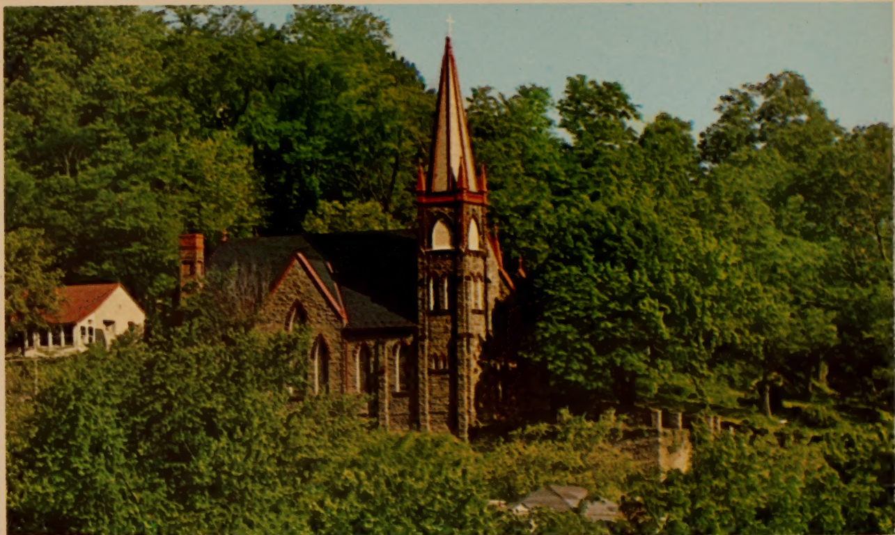
St. Peter's Catholic Church, Harpers Ferry, West Virginia
